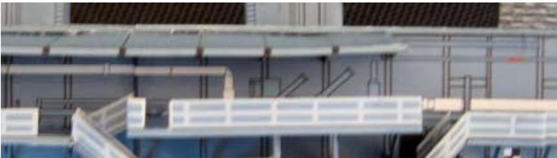
**Assembly of bottom deck (Crawler access)**
