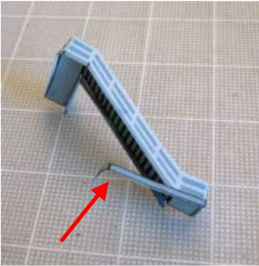
Extra beam that holds the stairway to the deck.
