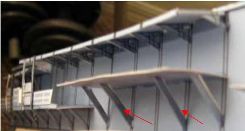
Note that the beams are different in size. The 2 in the middle are a bit larger than the rest for this deck.
